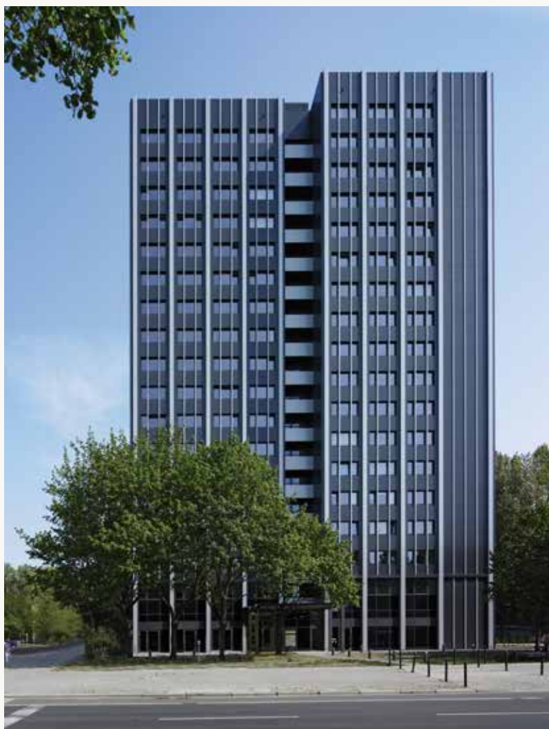
德国柏林弗里德里希斯海因的高层公寓楼翻新改造项目, 住宅楼, 2010年 Renovation of high-rise apartment buildings in Friedrichshagen, Berlin, Germany, Residential Project, 2010
