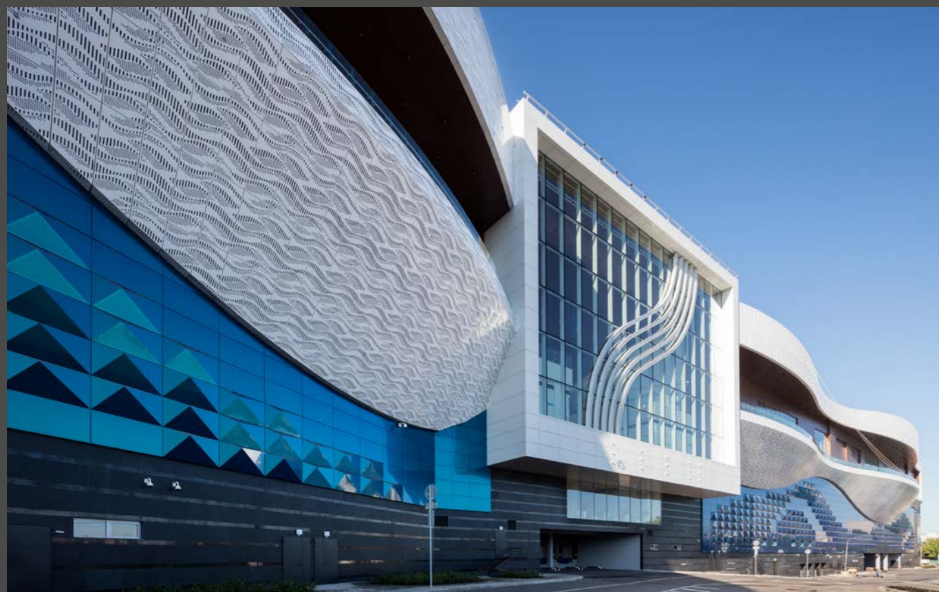
White perforated metal panels are placed alongside the blue | Perforiertes, weißes Metall rahmt das Blau ein.
