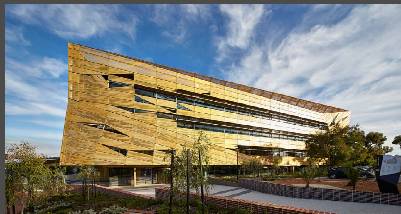
The combination of perforated aluminium and ALUCOBOND®. | Die Kombination aus gelochtem Aluminium und ALUCOBOND®
