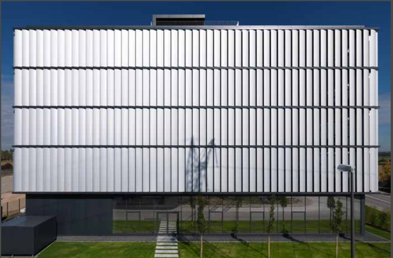
520 vertical, rotating aluminium louvre slats provide shade from the sun and can be either operated individually or centrally regulated. All photos: Richie Müller, Munich | 520 vertikale, drehbare Lamellen aus Aluminium bieten wahlweise individuell oder zentralgesteuerten Sonnenschutz.
